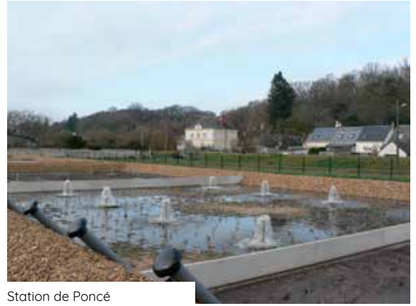
Station de Poncé
